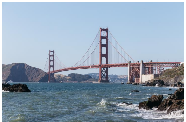
Golden Gate Bridge, San Francisco
